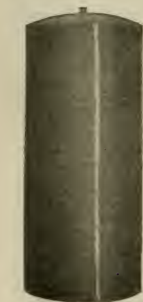
STEAM WELDED BY ELECTRIC ARC IN COMPRESSED AIR TANK.
